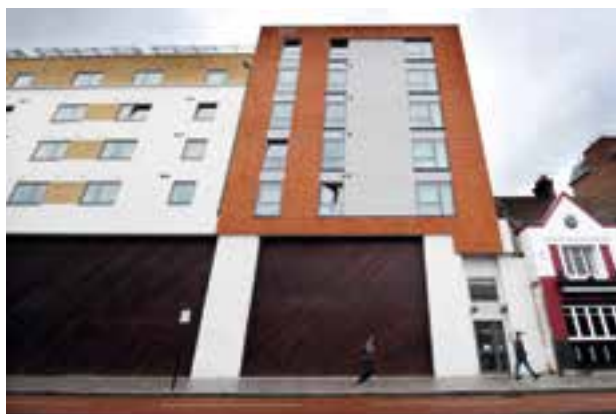
Image: Shared ownership housing scheme on Uxbridge Road in Ealing, London.
